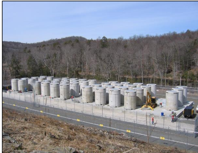
FIGURE 2. 2: SPENT FUEL STORAGE, CONNECTICUT YANKEE
